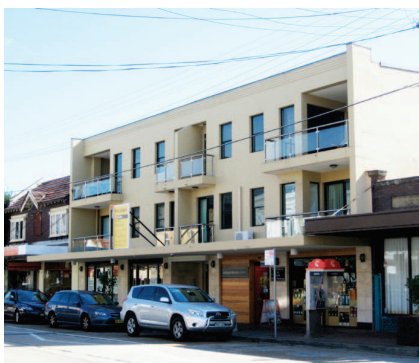
Figure 25 - Macpherson Street Bronte. Existing 3 storey infill building
